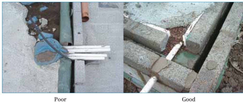
Figure 6. Examples of barrier installations
